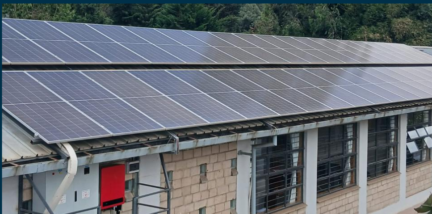
3. CEMESTEA SOLAR INSTALLATION
