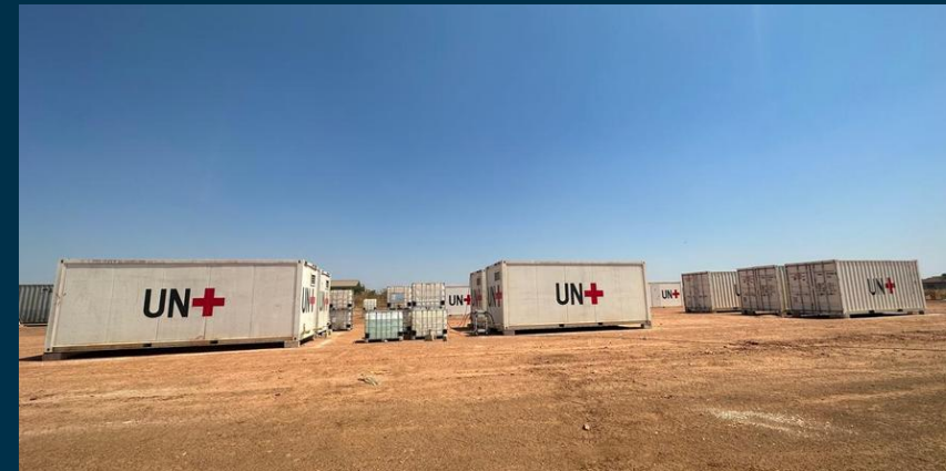
5. ZAMBIA - MINISTRY OF DEFENCE, UN MOBILE HOSPITAL SOLARIZATION
